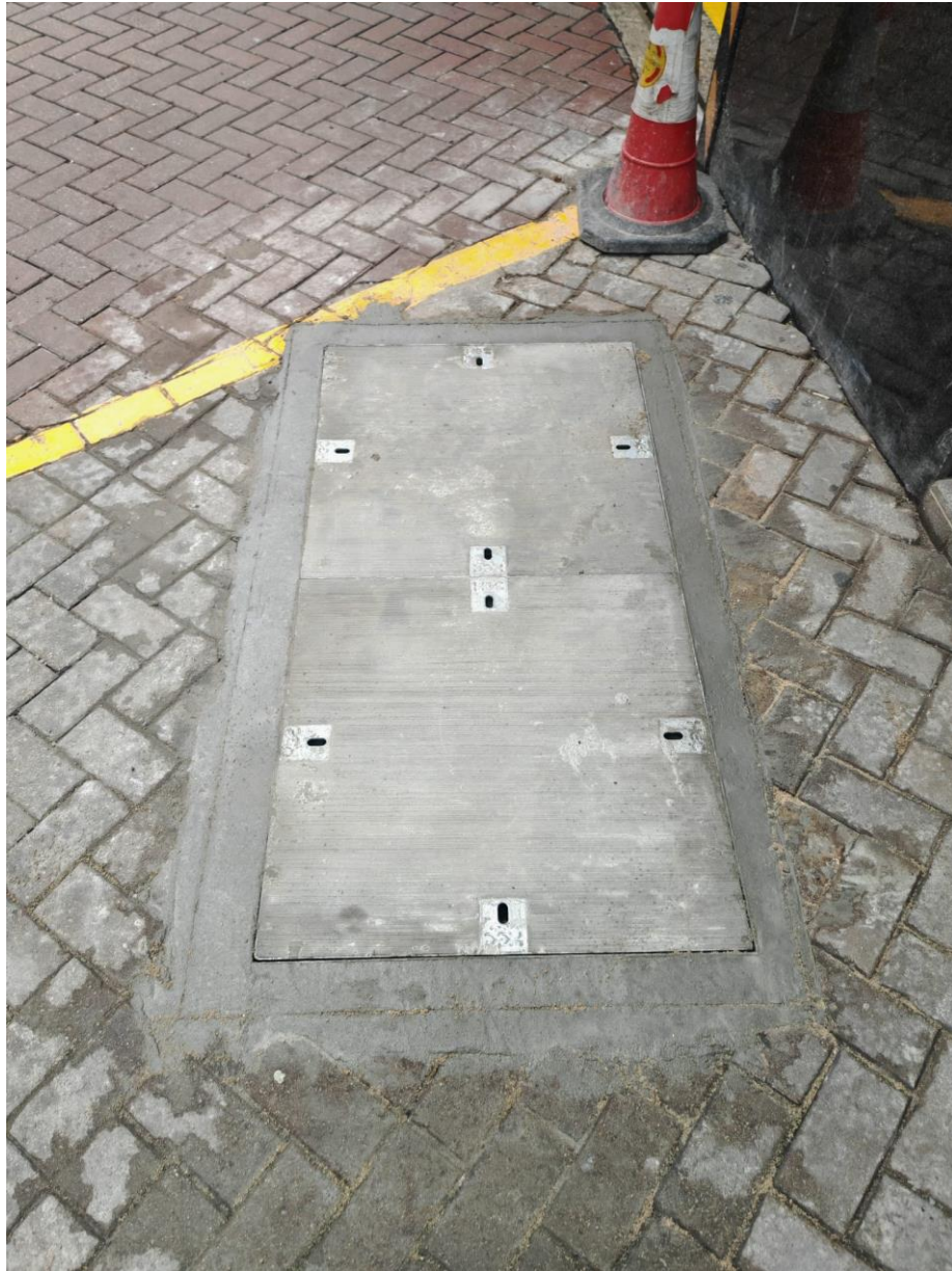
Photo for HGC's joint box with concrete cover - 2 pieces type at footway/cycle track with company logo "HGC"
