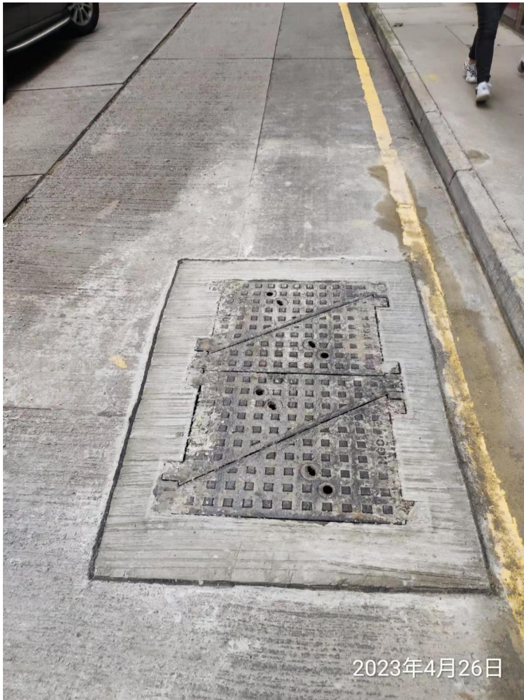
Photo for HGC's joint box with heavy duty cover - 4 pieces type at carriageway with company logo "HGC"
